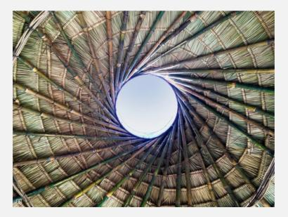
Smaller outbuildings provide a block making shelter, biogas-toilet with a reciprocal spiral bamboo roof topped by a repurposed metal drum rooflight, a thatched chicken roosting house, water catchment and filtration system, and a curved lattice split bamboo tunnel planted with native plants such as cucumbers and long beans. Hand painted stone signs in Khmer and English identify each building within the site.
